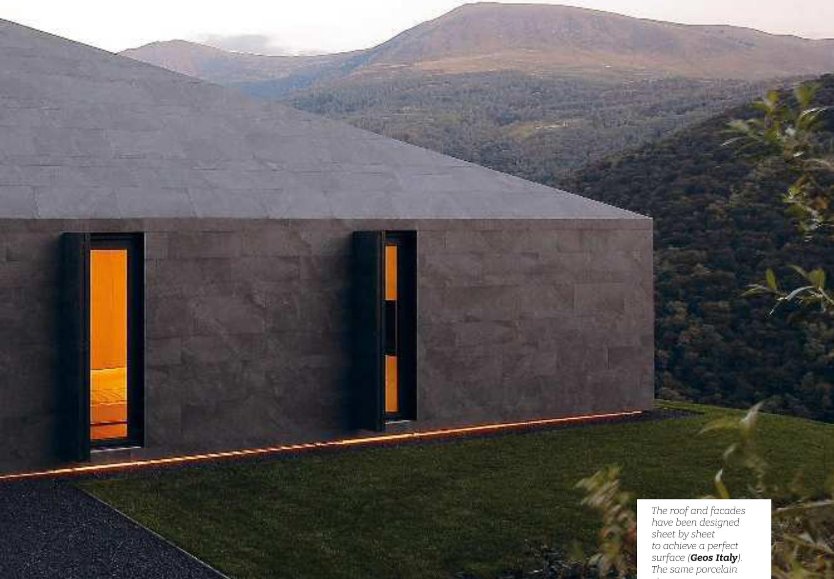
The roof and facades have been designed sheet by sheet to achieve a perfect surface (**Geos Italy**). The same porcelain stoneware (**Casalgrande Padana**) has also been used on the shutters, which when closed (small photo, left) completely vanish into the ceramic pattern. Below, section of the villa.
